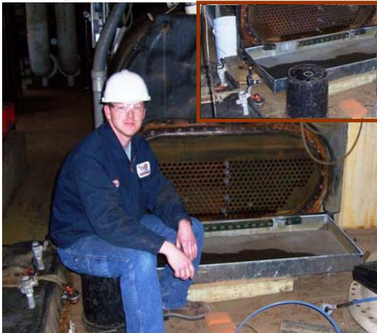
One of our Service HVAC Technicians did just that when he made a pan to collect water & debris from the chiller bundle that is being cleaned at Schlitz Park. A hose is attached to the pan to safely direct the waste away from the work area. In the past, all the water & sludge from inside the chillers would be on the floor causing a mess to clean up and creating a safety hazard. This pan, shown in the picture at left, was an easy solution to a messy problem.
